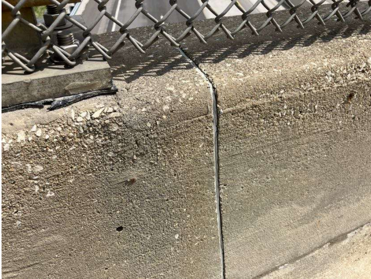
PHOTO 4 View of typical joint on parapet wall. Samples taken of caulk material.
