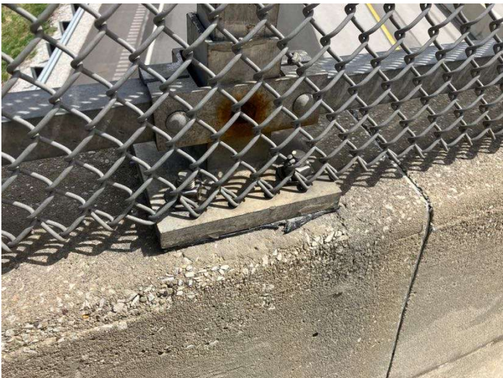
PHOTO 6 View of the vandal fence base plate. Samples taken of caulk material.
