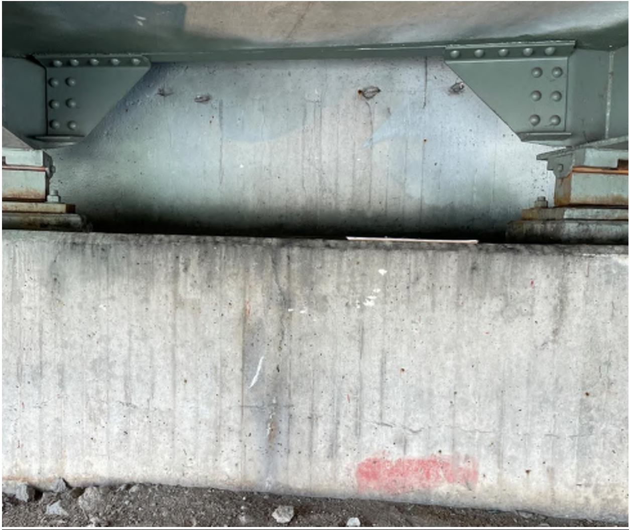
Photograph #8 - Forward (North) Abutment Vertical Crack MP 182.1
