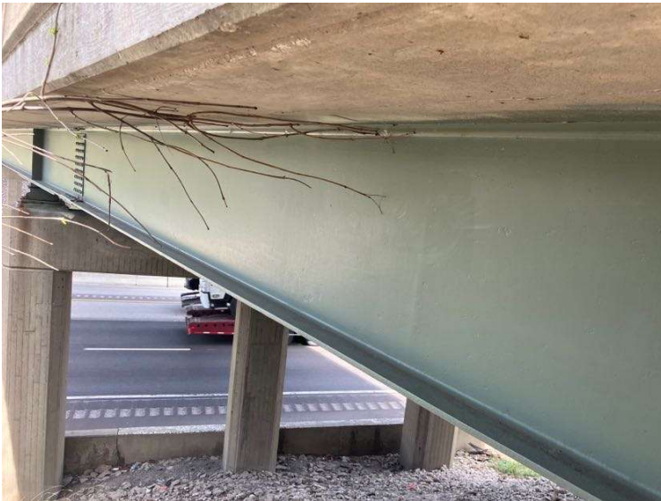
PHOTO 5 View of outer beam. Paint in good condition.
