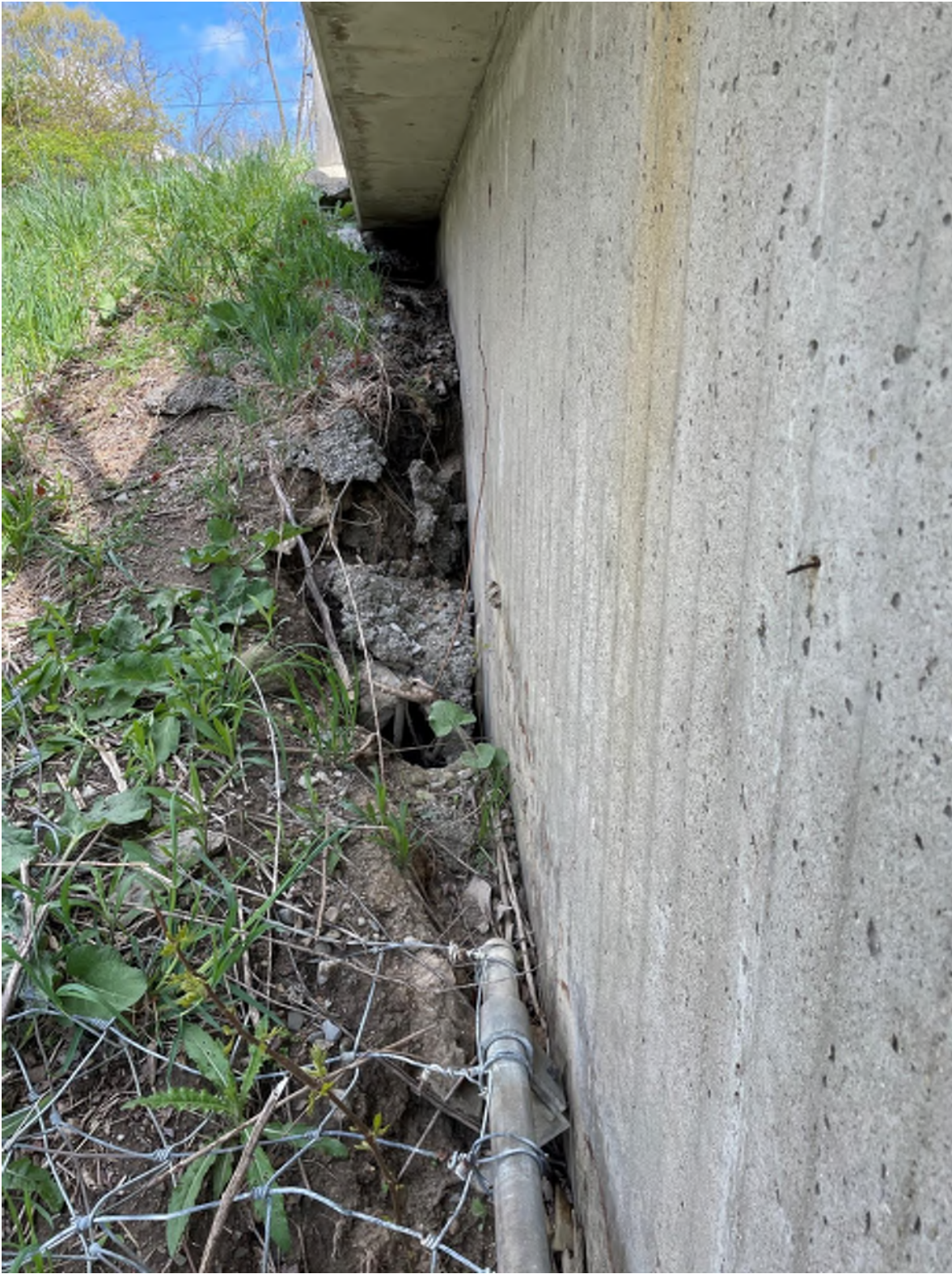
Photograph #10 - Typical Wingwall Condition and Slope Erosion at Forward Left (Northwest) MP 182.1
