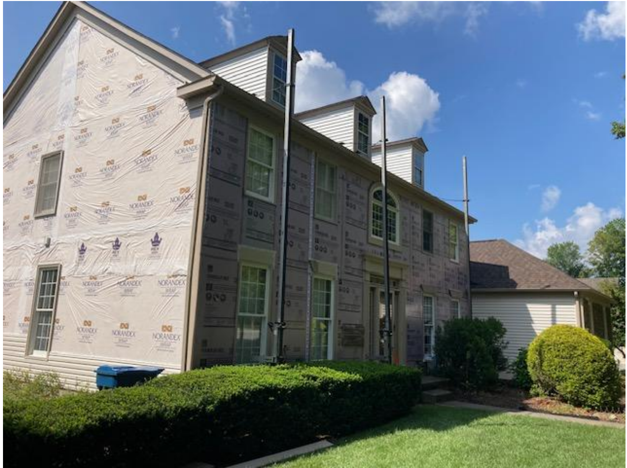
East side transition to North side: Vertical trim board upgraded from wood to wood-grained AZEK of the same color.
