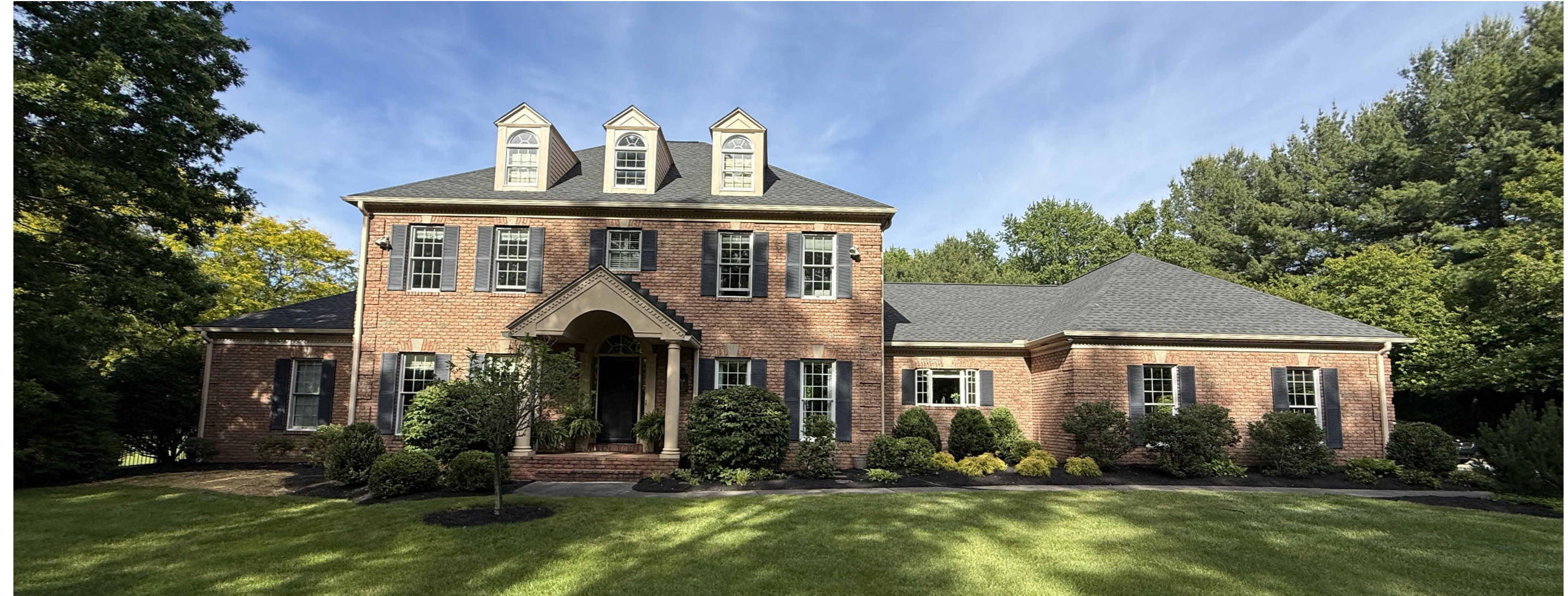
EXISTING FRONT FACADE
