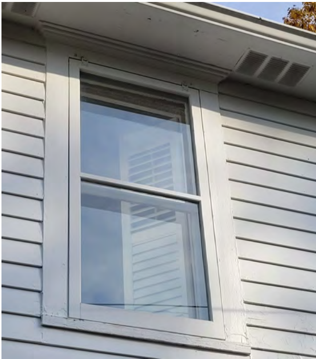
Image 3: Detail view of a typical presumed historic second-floor wood window. Note the window with presumed historic storm window trim and how it differs from the first-floor historic wood window.
