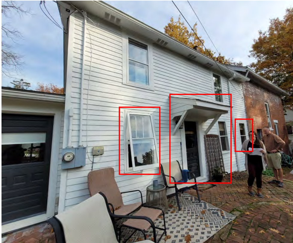
Image 1: Rear (west) elevation. The red boxes indicate the historic wood windows and non-historic wood door in presumed historic location/opening with non-historic shed roof overhang to be removed.
