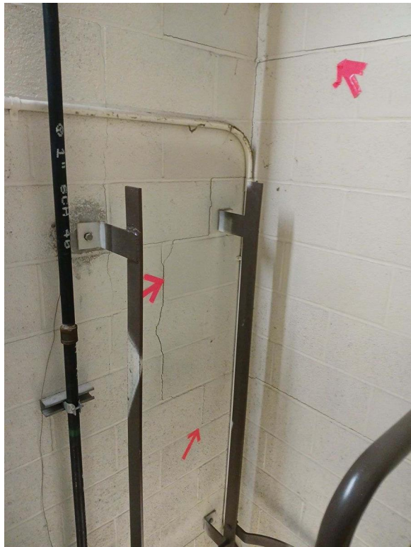
HOSE TOWER SETTLEMENT CRACKS
