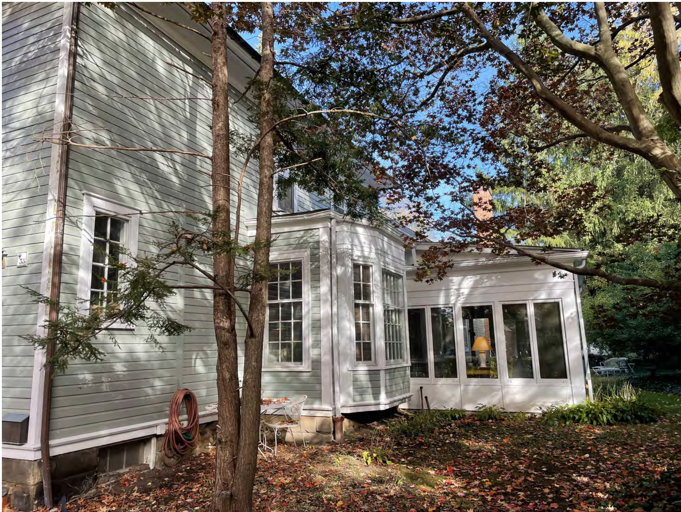
SOUTH ELEVATION - FROM FRONT YARD
