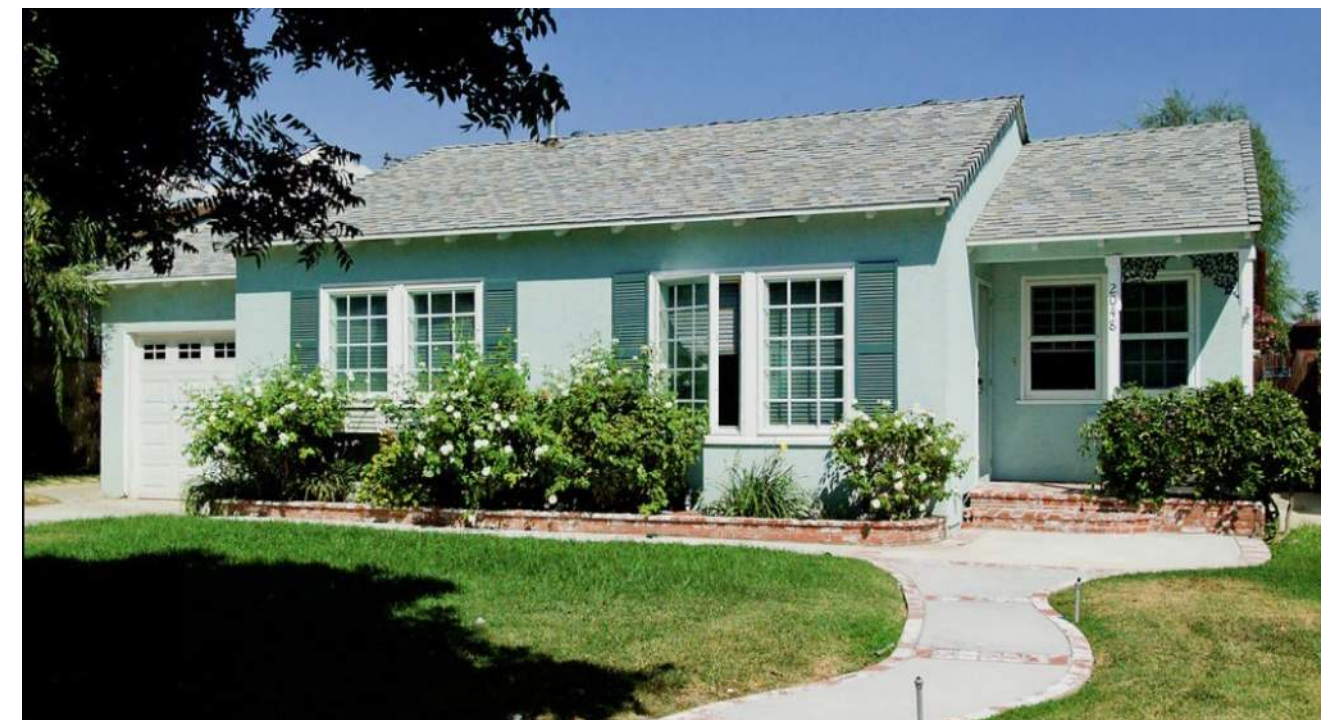
SIDE-GABLED ROOF (CAPE COD); MINIMAL TRADITIONAL Burbank, California; 1941 (renovated 1953). Windows on the main house block are not double-hung and are likely later additions.
