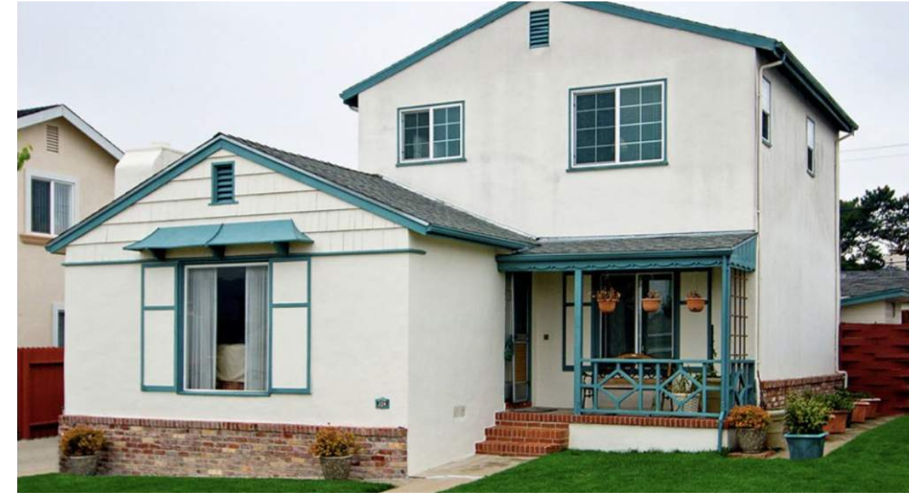
GABLE-AND-WING ROOF; MINIMAL TRADITIONAL South San Francisco, California; ca. 1940s. Compare to the following example in the same area. The second-story gable could be original or an addition. The window in the first-floor gable appears modified.
