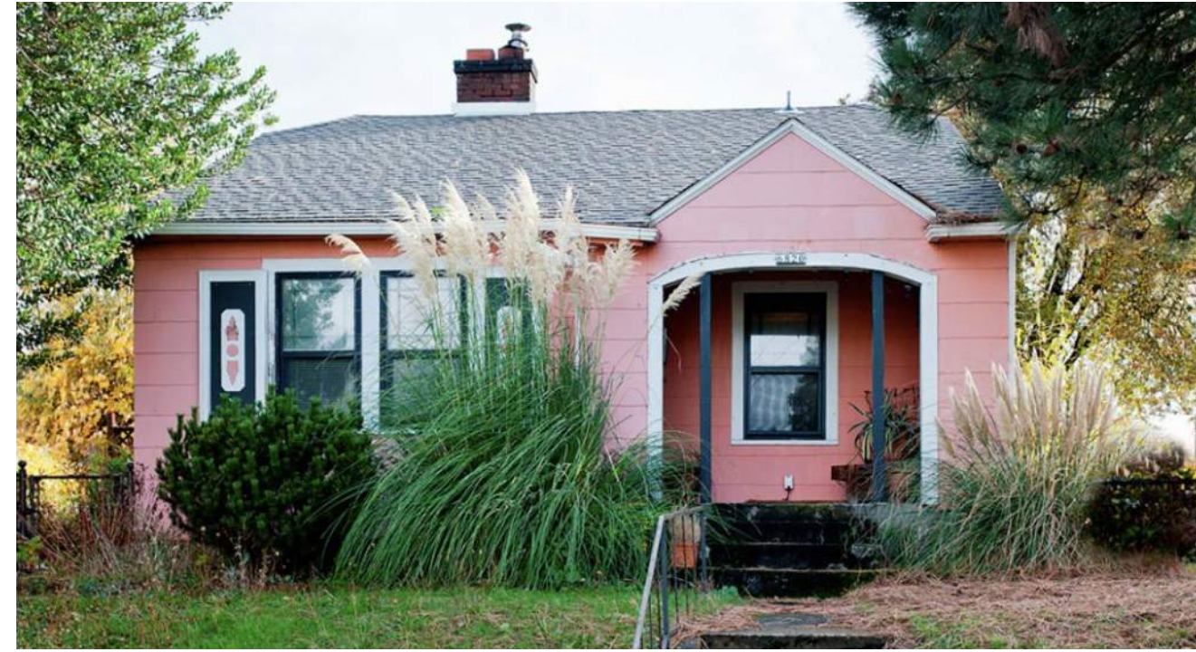
GABLE-AND-WING ROOF; MINIMAL TRADITIONAL Portland, Oregon; ca. 1930. This early example is unusual in having the entry in the gable.
