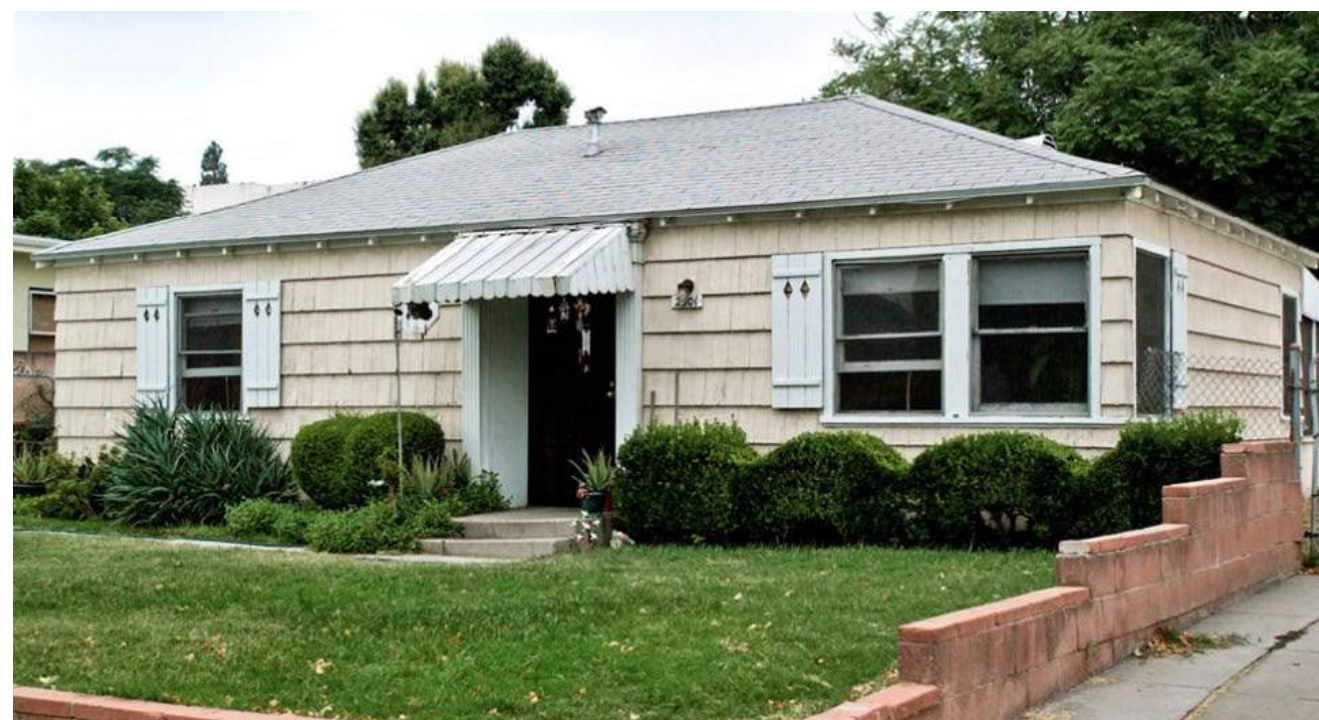
OTHER ROOF; MINIMAL TRADITIONAL Burbank, California; ca. 1940. Note the shingle cladding, and board shutters with cutouts (even on corner windows).
