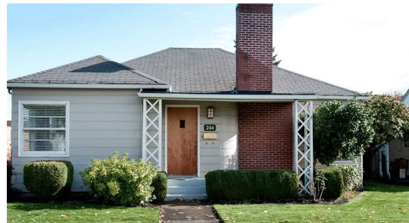
OTHER ROOF; MINIMAL TRADITIONAL Portland, Oregon; ca. 1940s. The corner-window placement was among the FHA's recommended designs.
