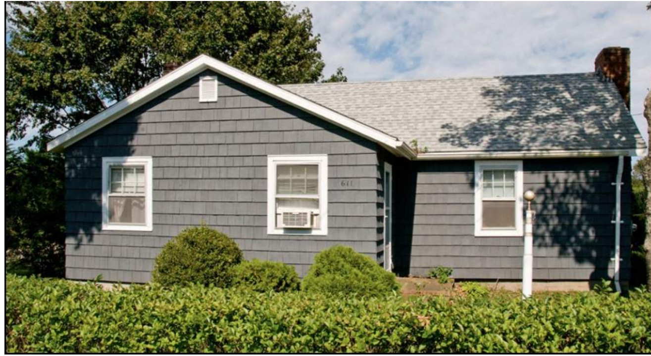
GABLE-AND-WING ROOF; MINIMAL TRADITIONAL Hamptons, New York; ca. 1940s. Note the double-hung windows and overall cladding. Door faces to side.
