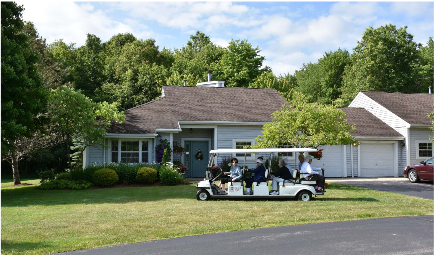
BELOW: Original Villas 1-58 with 1-car garages
