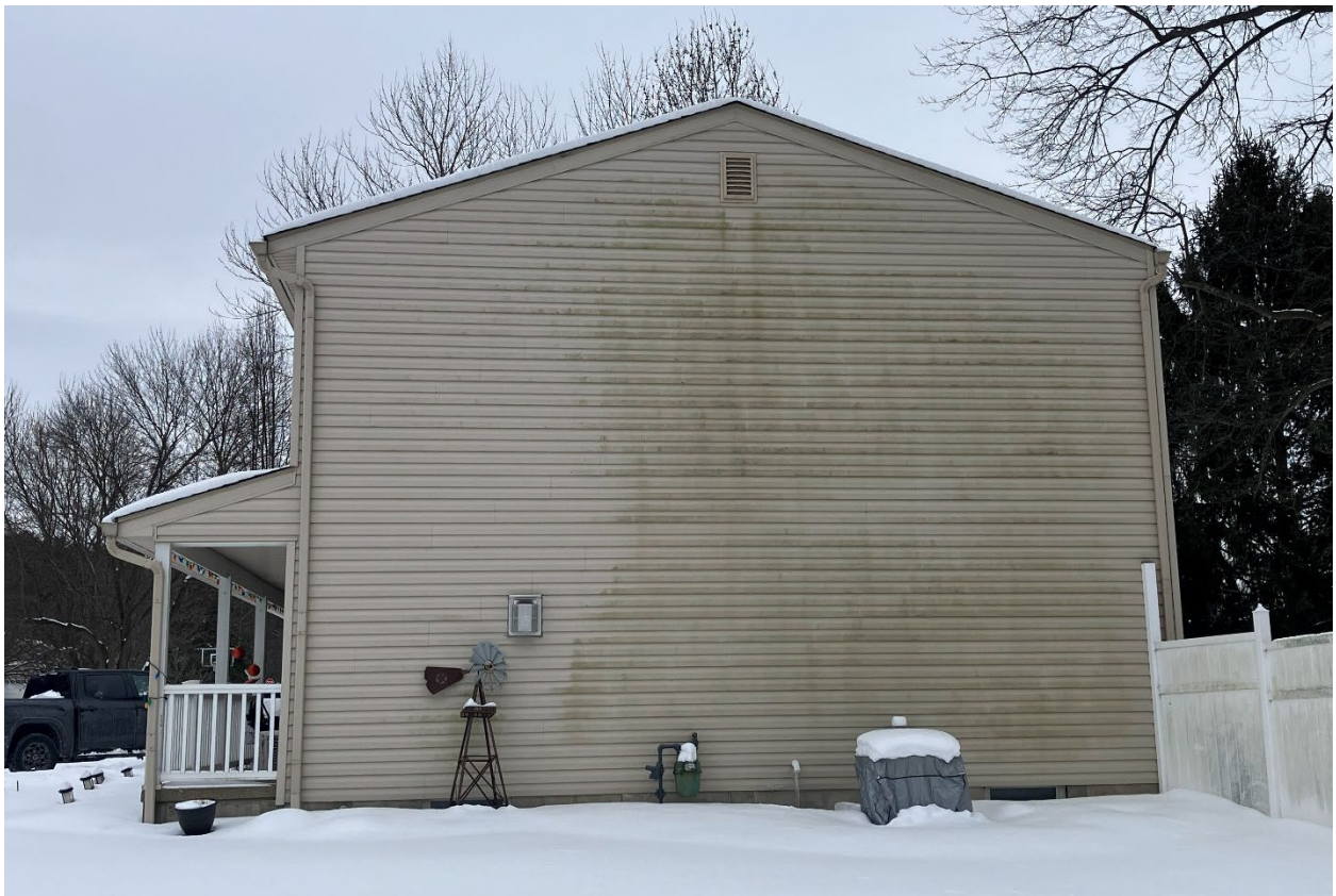
Overall photo of west elevation of where the new addition is proposed.
