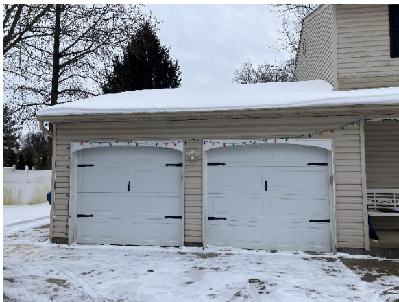
Close up of the existing garage.
