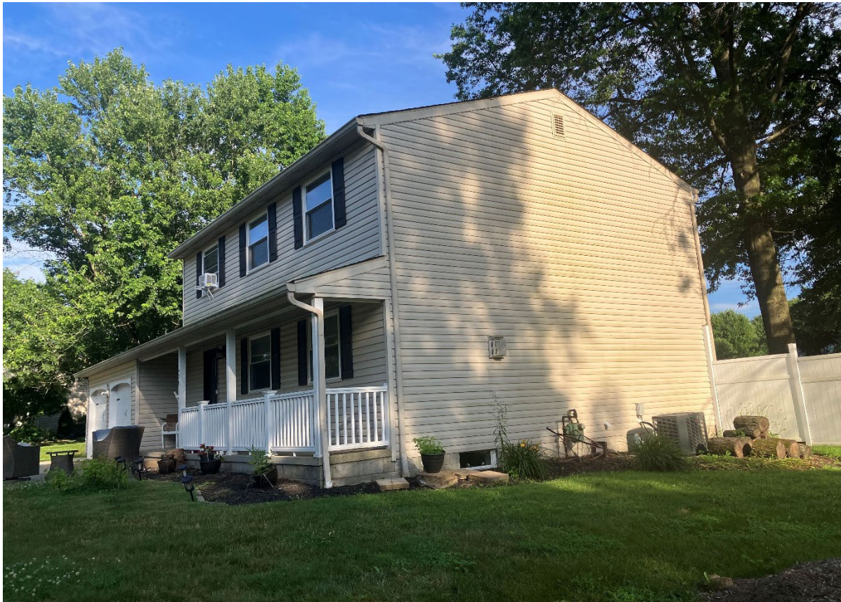
Northwest corner of the residence and location where the addition is proposed.
