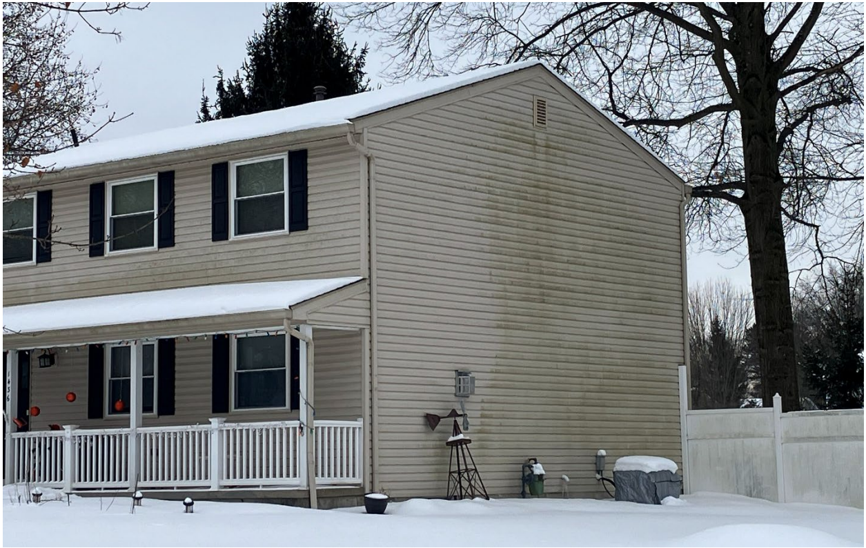
Additional view of Northwest corner and location where the addition is proposed.
