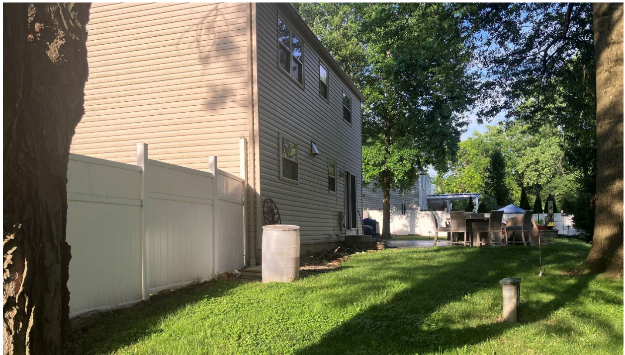
Backyard and backside of the existing main structure.
