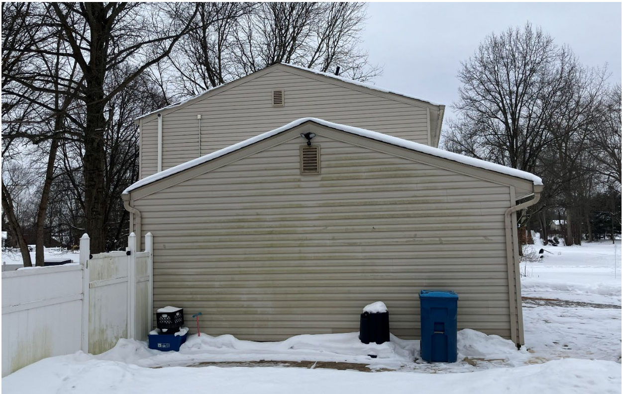
East elevation and side of the existing garage, with the main building beyond.
