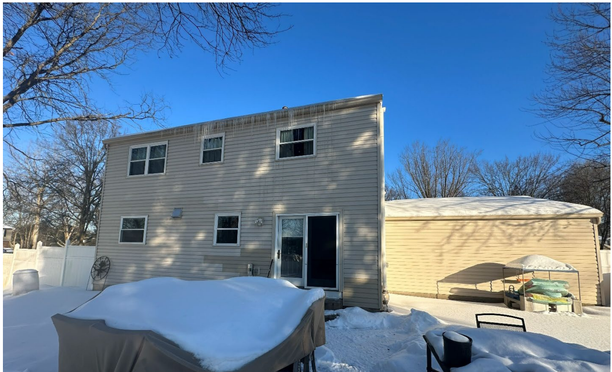
Backside of the existing main structure.
