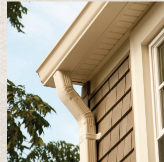
Rainware, Fascia, Soffit
