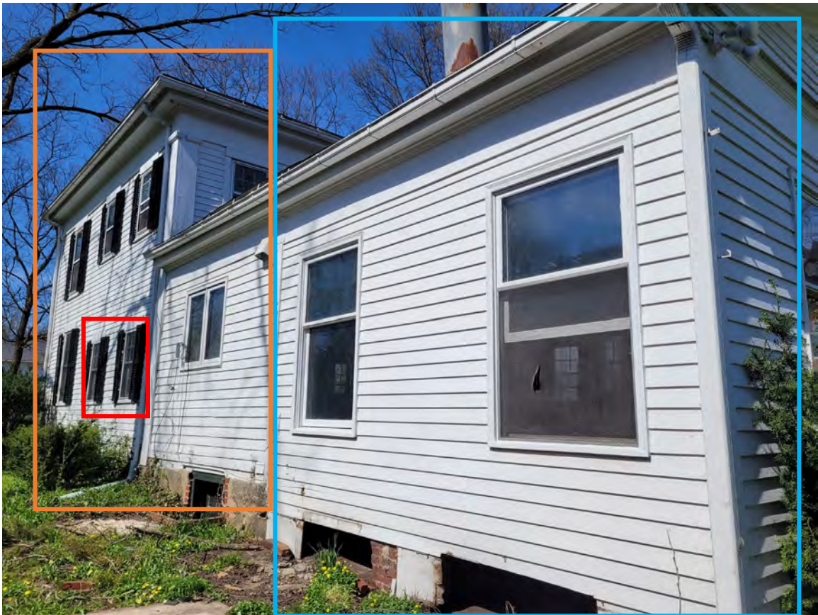
Image 7: Side (west) elevation. The orange block indicates the 1913 addition. The green box indicates the 1925 addition. The blue boxes indicates an addition with an unknown date. The red boxes indicate the vinyl replacement windows.
