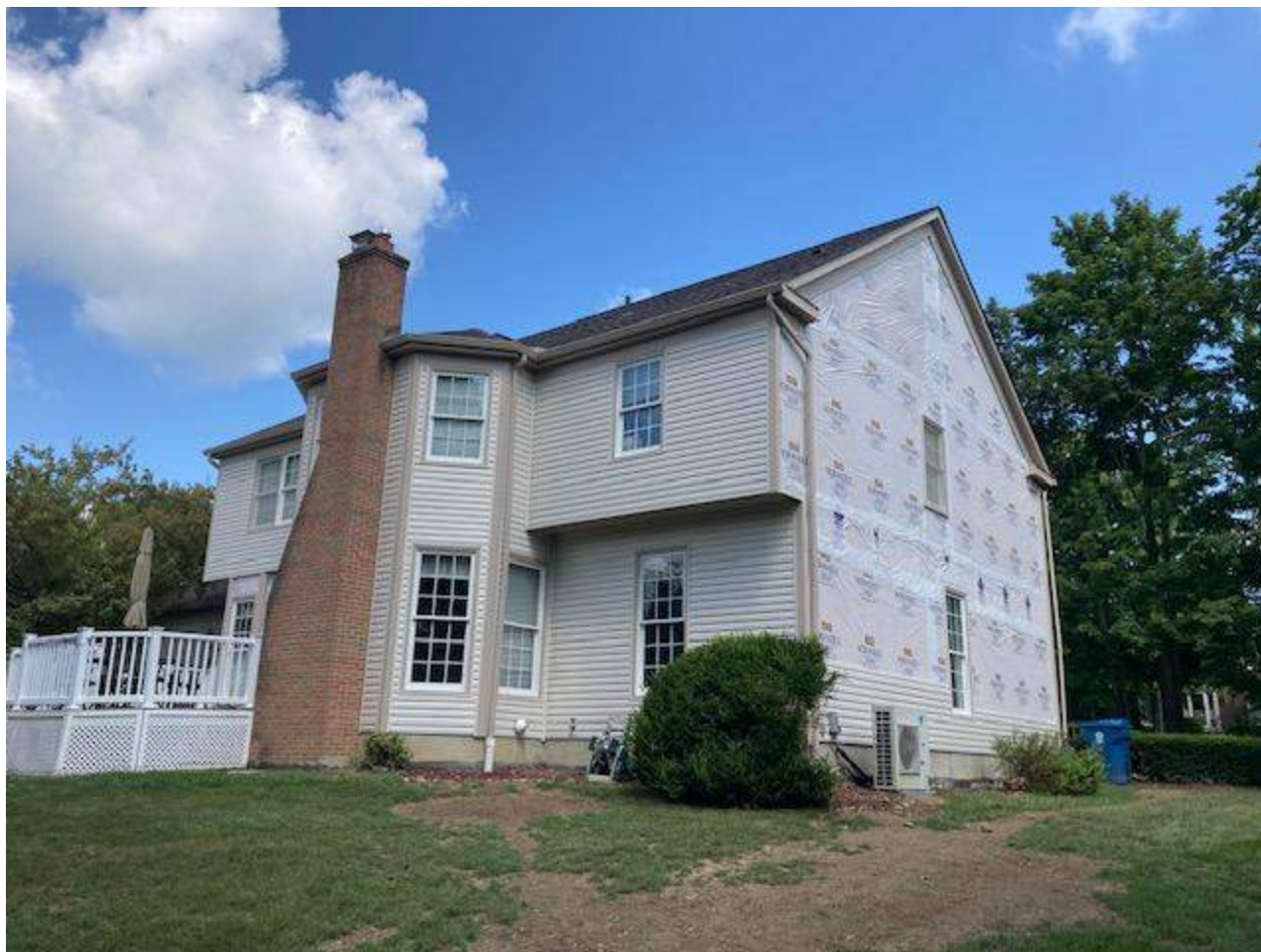
South side transition to East side: Corner posts upgraded from wood to wood-grained AZEK of the same color.
