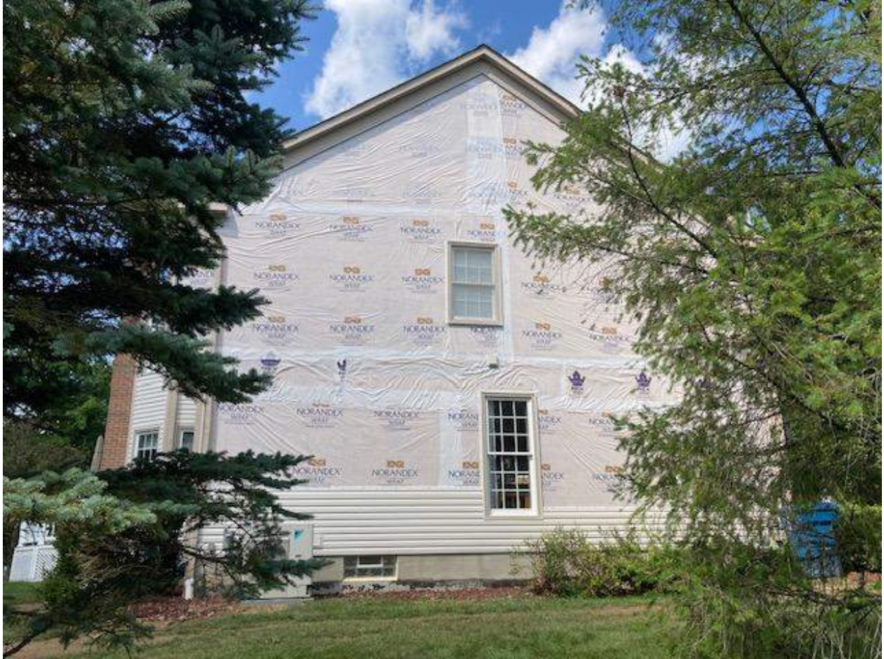
East side: Aluminum siding replaced with insulated vinyl siding of same style and color. Frieze boards upgraded from wood to wood-grained AZEK of same color.
