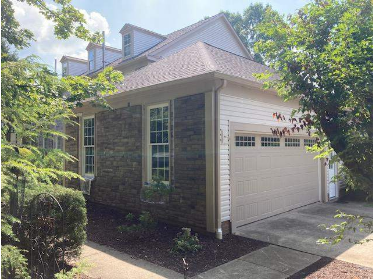
North side transition to West side: Corner posts upgraded from wood to wood-grained AZEK of same color.
