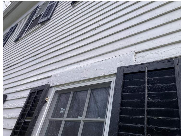
THE EXISTING SIDING, SHUTTERS AND TRIM HAVE DETERIORATED BEYOND REPAIR:
