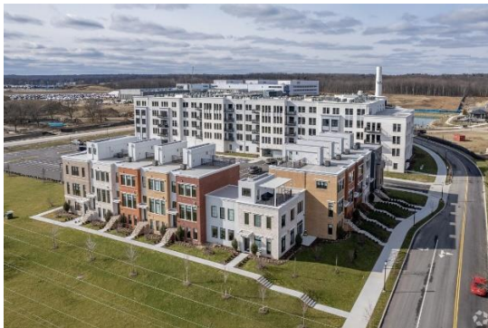
Transition from three-story townhomes, five-story apartment building and then commercial/industrial use.
