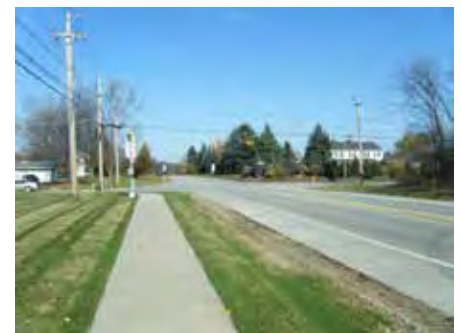
Sidewalk along Stow Road in front of Ellsworth Hill Elementary
