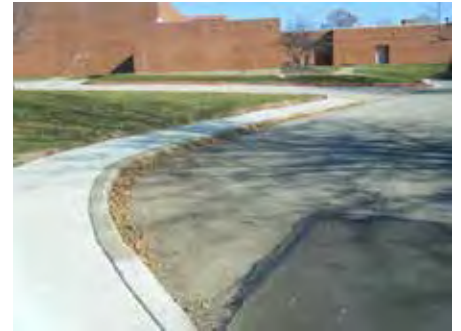
New sidewalks constructed near the Natatorium at East Woods Elementary
