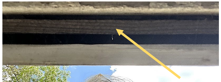
View from below at the foundation, looking upwards underneath the aluminum siding, showing historic wood siding
