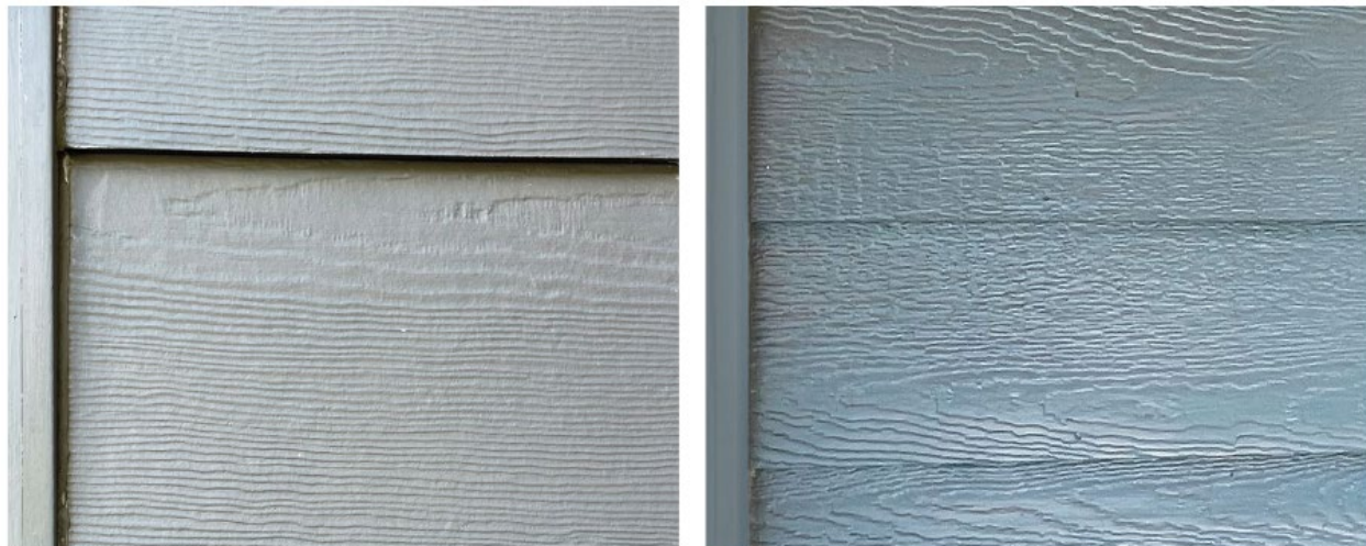
Figure 14. Surface texture is an important aspect in matching the appearance of a historic material, especially when a material is viewed at close range. As seen in these two images, many of the substitute materials produced for siding and trim have an embossed wood grain, making them incompatible for replacing historic wood that was typically planed to a smooth surface. Some substitute products are available with a smooth surface as well. Photos: John Sandor, NPS.
