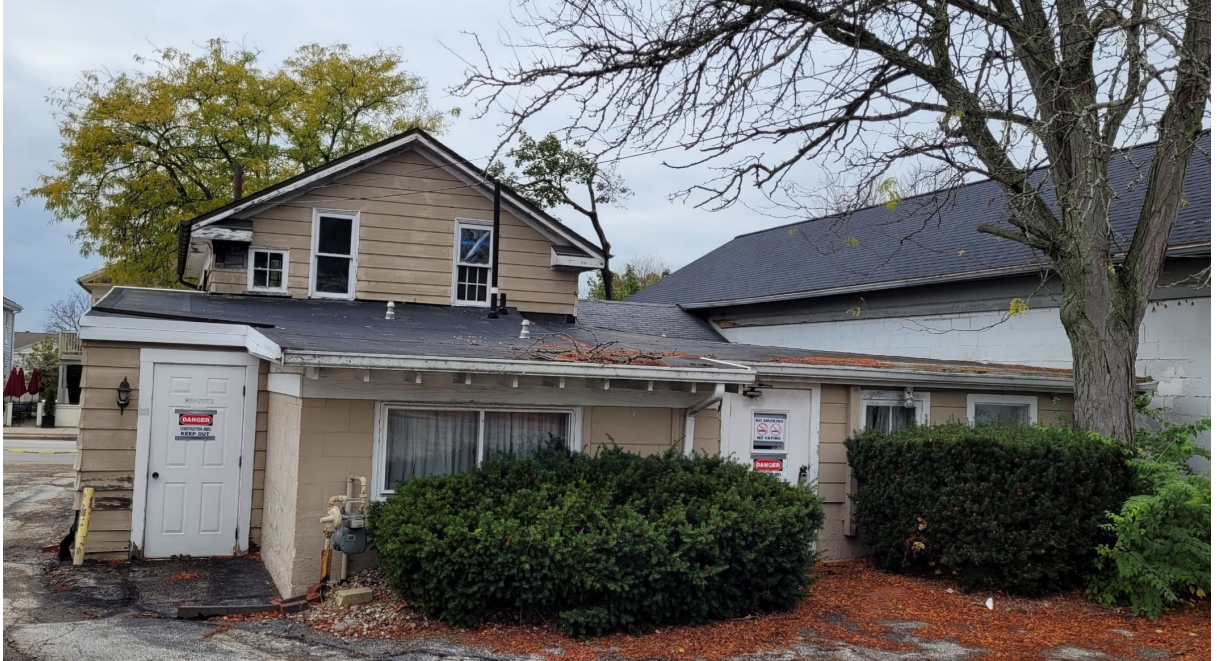
Image 8: Rear (east) elevation. One-story rear addition to be removed, including presumed addition that existed by 1916 according to the Sanborn map in Image 3.
