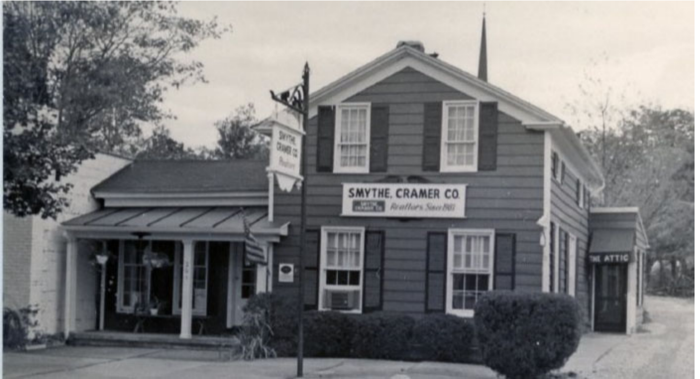
Image 6: Date c.1970. Courtesy of the Hudson Historical Society. This is the presumed configuration from the 1954 restoration. Front (west) elevation. Note the front porch reconfiguration, the window replacements on the two-story portion, the replaced windows at the porch, and the one-story rear addition.
