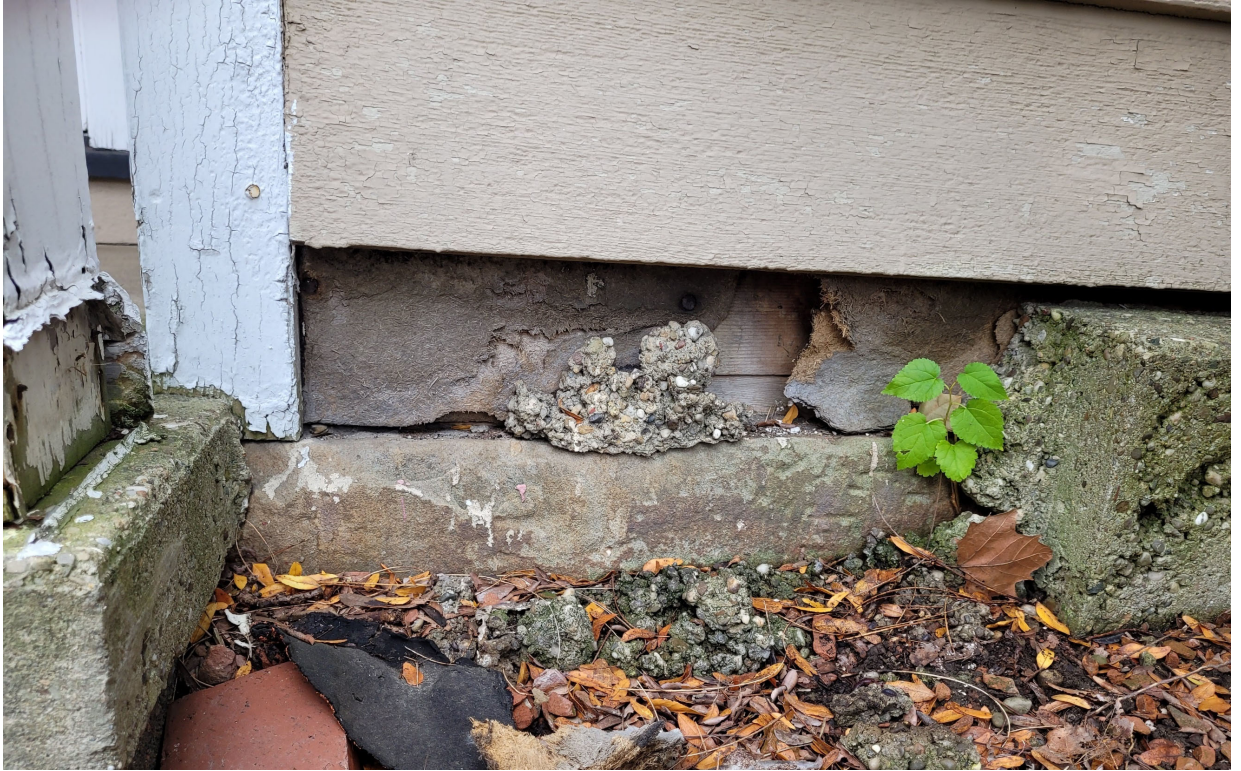
Image 10: Front (west) elevation. Detail at two-story portion showing sandstone foundation behind concrete. Also note wood siding behind the existing siding and mineral wool.
