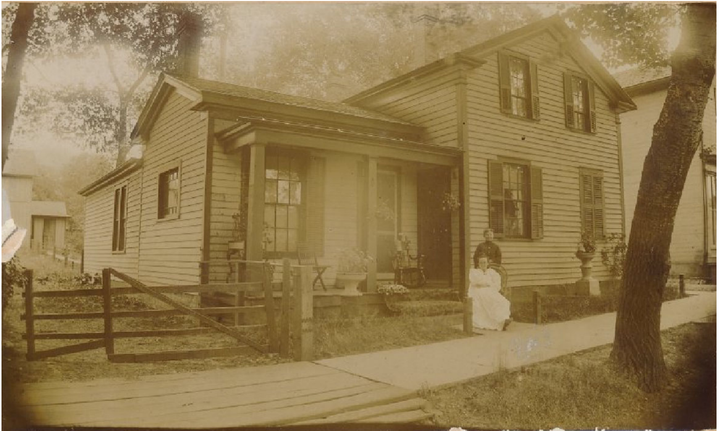
Image 1: Date c.1900. Courtesy of the Hudson Historical Society. Front (west) and side (north) elevation. Note the Gable-Front-and-Wing configuration of the house, the 6 over 6 double hung windows on the first floor, the exposure width of the siding, the two chimneys appear to be brick, and the foundation appears to be stone. The door appears to be under the porch on the north return wall.
