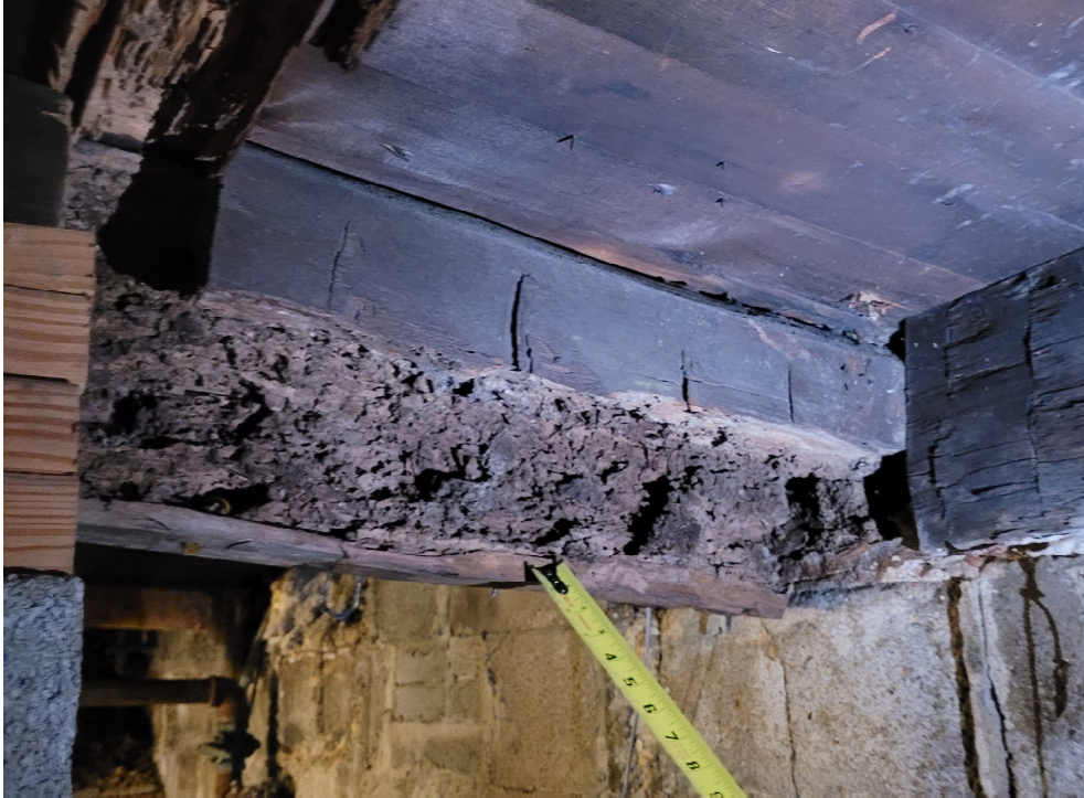
Image 12: Image taken in basement showing termite damage to the north-south structural member in the two-story portion.
