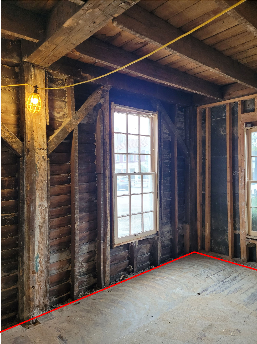
Image 11: Interior, southwest corner of the two-story structure. Red line indicates where structure will be cut to be lifted.
