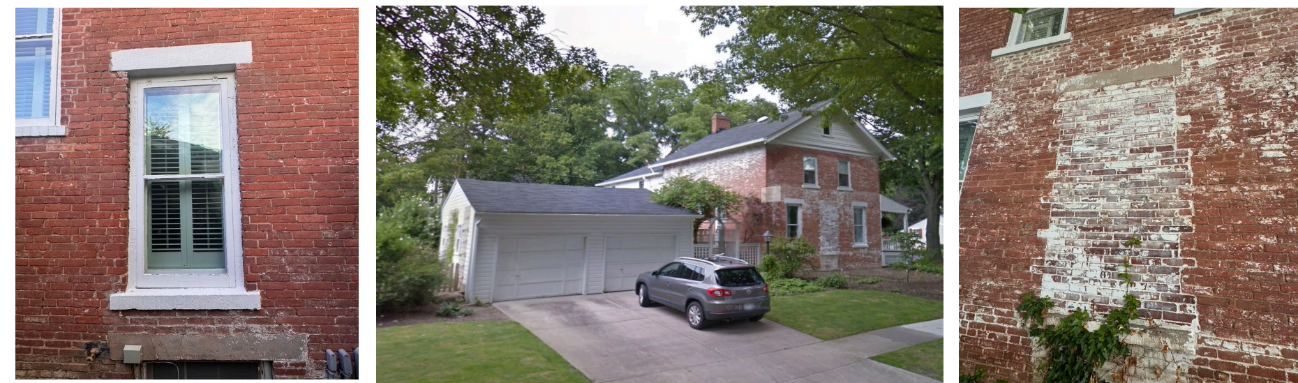
EXISTING HOME DETAILS REPEATED IN THE FIREPLACE
