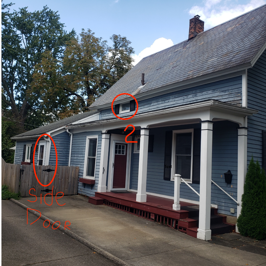
Left side of the house. Replacing 1 window and side door.
