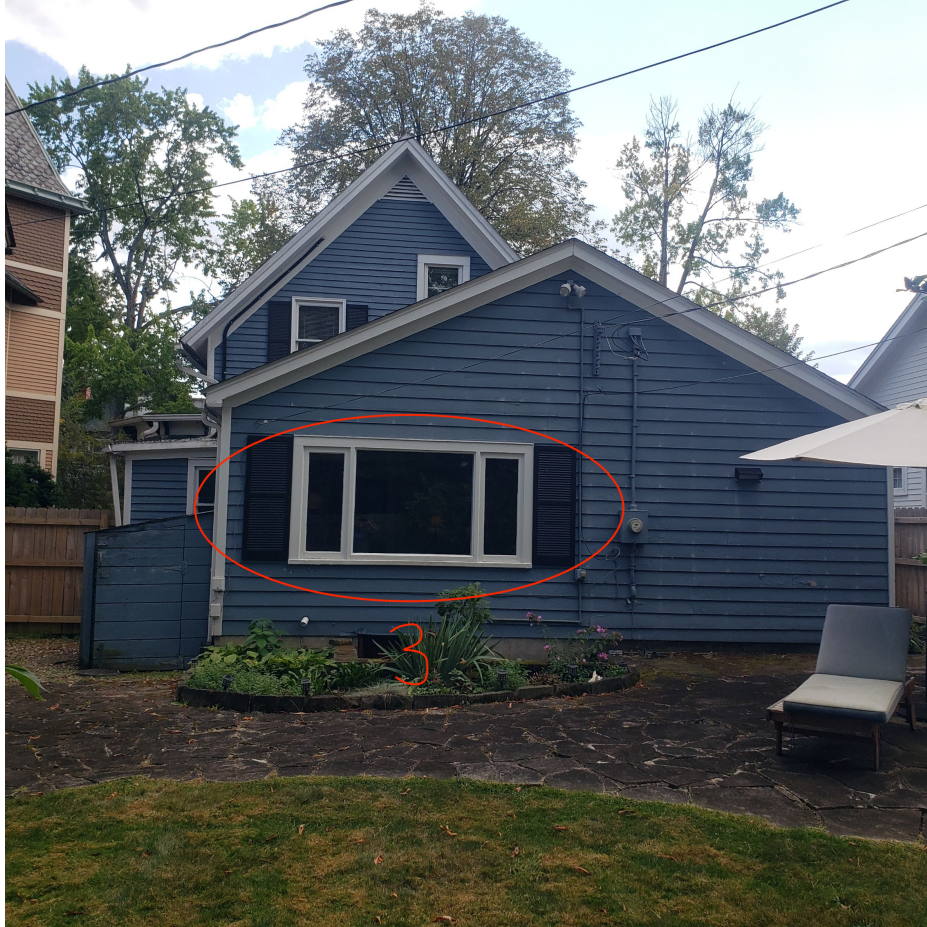
Back side of the house. Replacing 3 section window.
