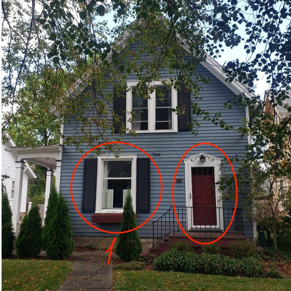
Front of the house. Replacing 1 window and front door.
