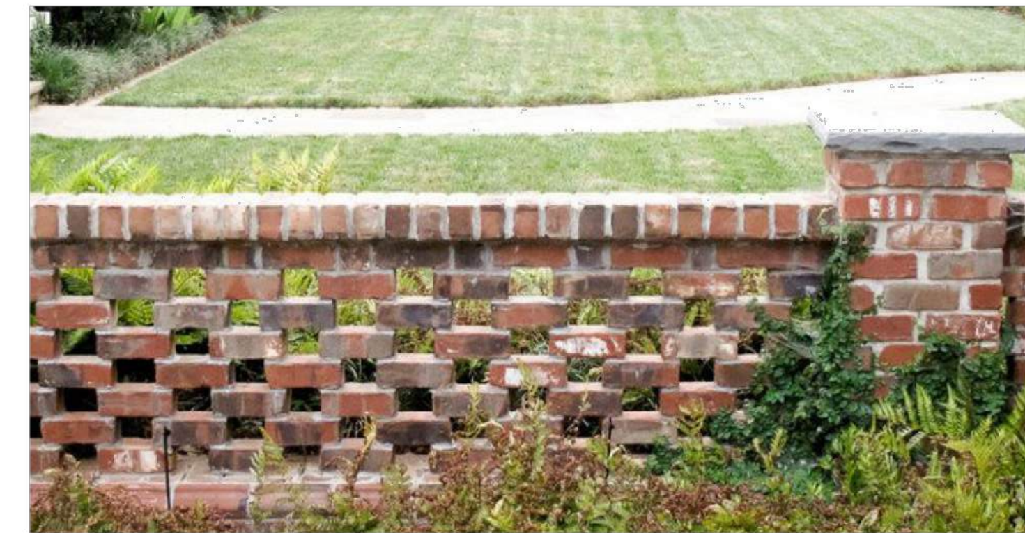
Perimeter Wall - Window into Park
