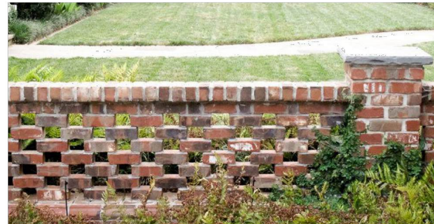
Perimeter Wall - Window into Park
