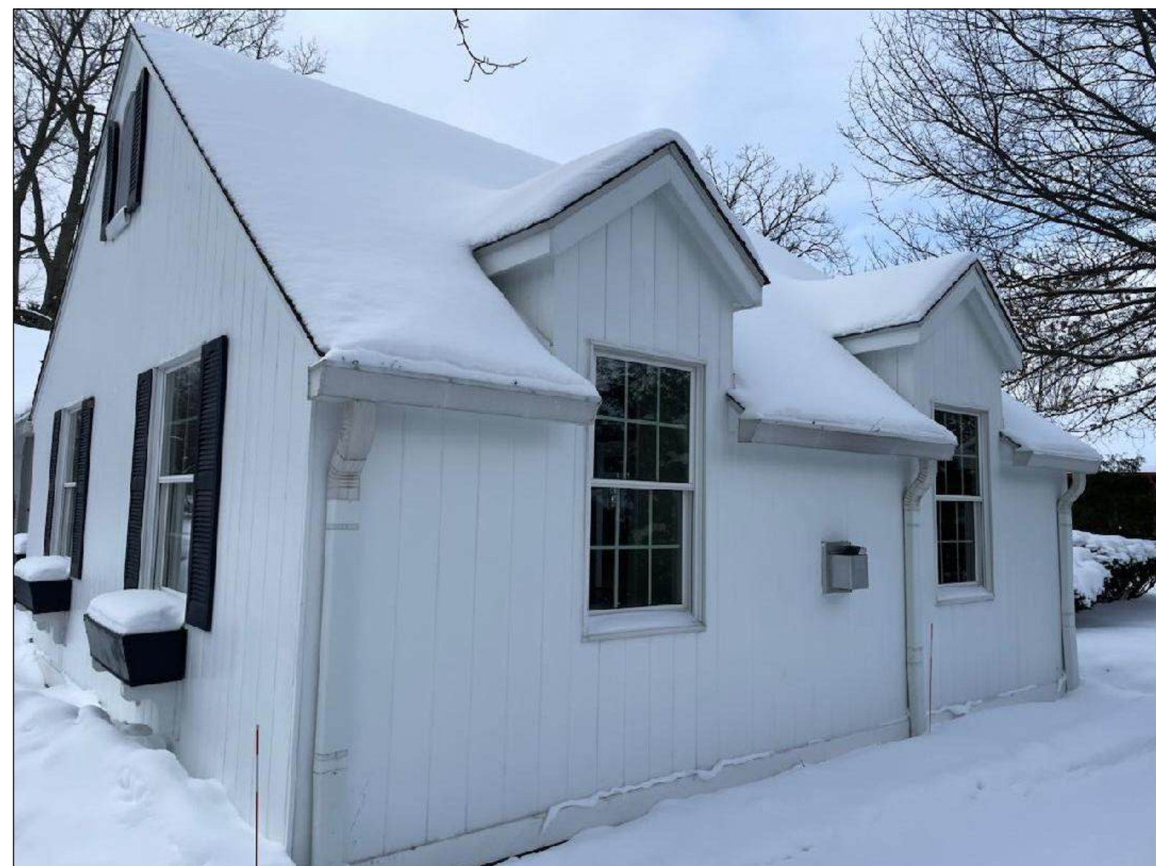
existing house - front s.e. corner
