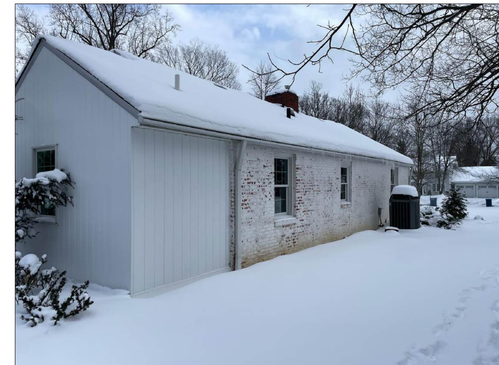
existing house - rear n.w. corner
